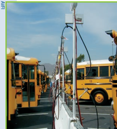
Time-fill pumps fuel vehicles over a longer period of time—usually overnight.
