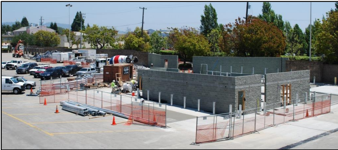
Figure 5. Construction progress on the Emeryville hydrogen fueling station
