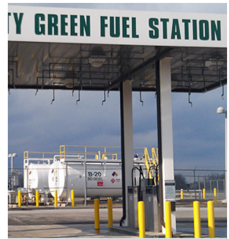
Through its portfolio of green projects, the Atlantic County Utilities Authority has significantly reduced its greenhouse gas emissions and saved more than $2 million a year in operating costs. Photo from Atlantic County Utilities Authority
