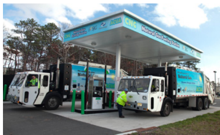
Through its portfolio of green projects, the Atlantic County Utilities Authority has significantly reduced its greenhouse gas emissions and saved more than $2 million a year in operating costs. Photo from Atlantic County Utilities Authority
