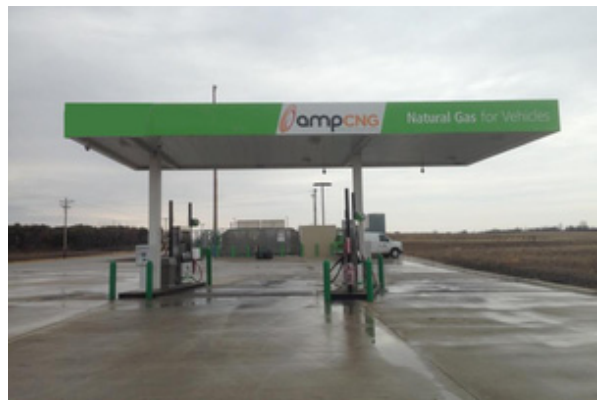
FIGURE 2 The ampCNG R-CNG refueling station at Fair Oaks. (Photo courtesy of ampCNG, http://www.ampcng.com/stations/ .)
