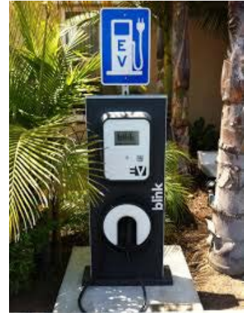
Photo 15. The connector on this EVSE unit is low to the ground to meet ADA accessibility requirements. Photo from Ecotality.
