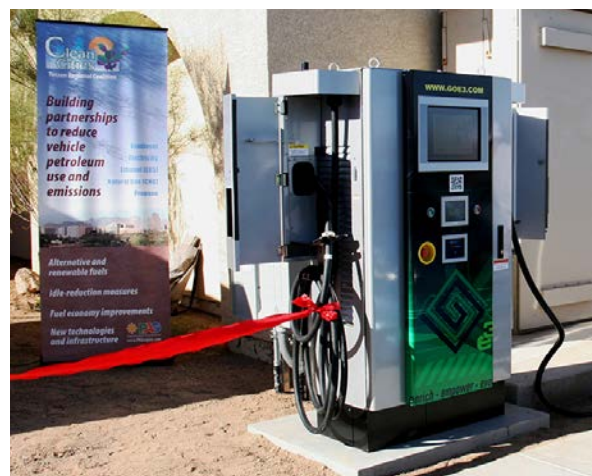
Photo 18. This DCFC unit is part of the Arizona EV Highway corridor project linking Tucson to Phoenix. Photo from Pima Association of Governments, NREL 24345.
