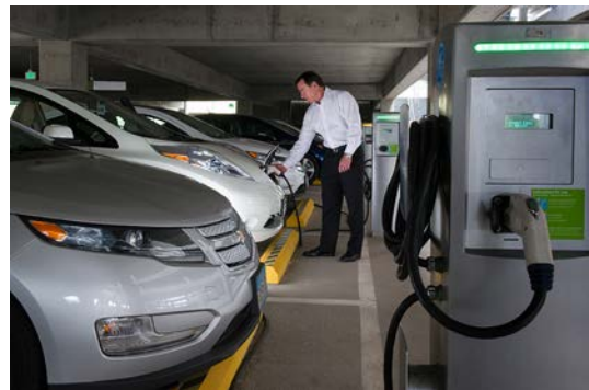
Photo 5. NREL employee plugging in his electric vehicle in one of the 36 EVSE in the NREL parking garage. Photo from Dennis Schroder/NREL, NREL 26675.
