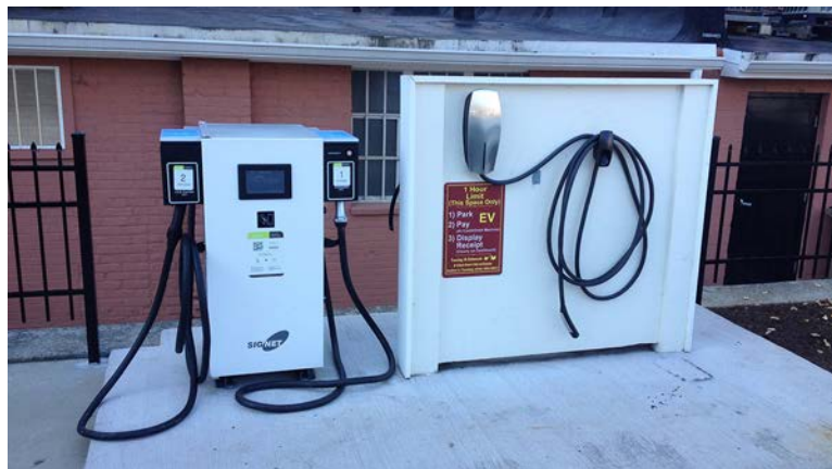
Photo 24. This public parking lot in Charlottesville, VA offers DC fast charging using SAEJ1772 CCS and CHAdeMO connector standards as well as a Tesla Level 2 connector. Photo from Margaret Smith.
