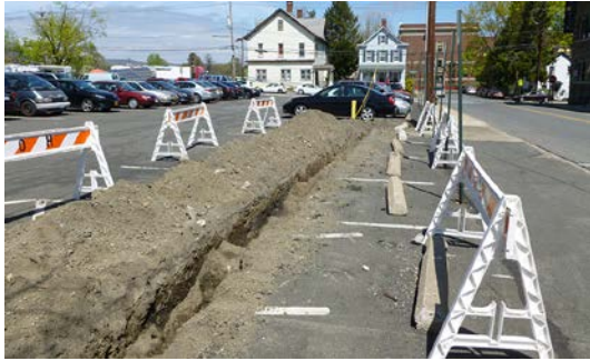
Photo 7. Trenching through a parking lot to install a public dual-port Level 2 EVSE in Haverstraw, N.Y. Photo from New York State Research and Development Authority (NYSERDA).
