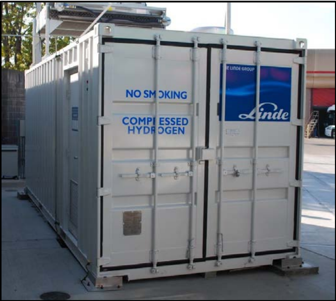
Figure 8. The Linde MF-90 high pressure compressor at the Emeryville station
