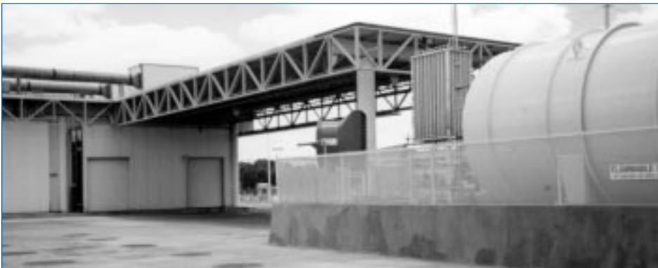
Figure 6. Northwest fueling station, showing canopy where fuel lines run from tank to fueling lanes
