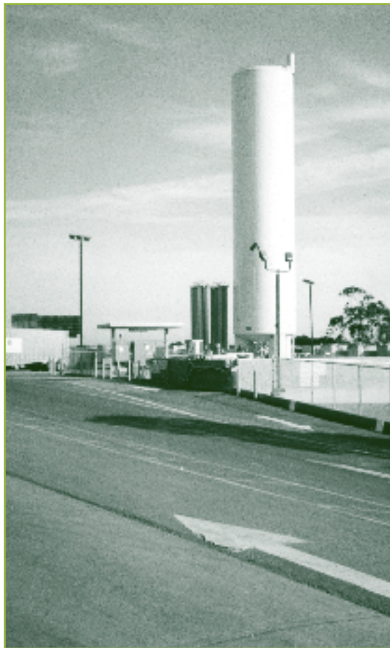
Figure 3. LNG Fueling Station at SF Recycling & Disposal
