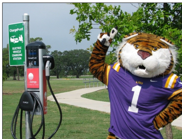
Charger installed on the Louisiana State University campus. Photo from Louisiana State University
