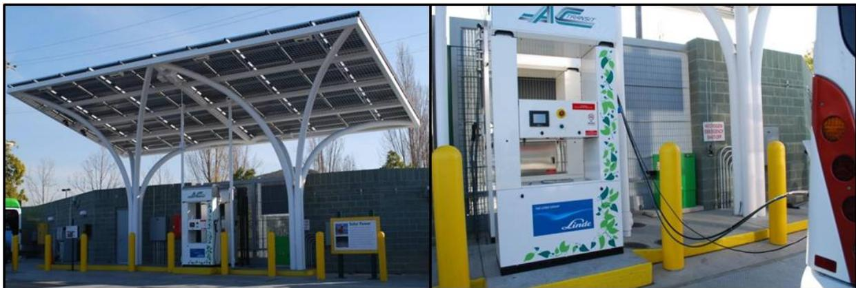
**Figure 7. Bus fueling at the Emeryville hydrogen station: fueling area (left) and close-up of the bus dispenser (right)**
