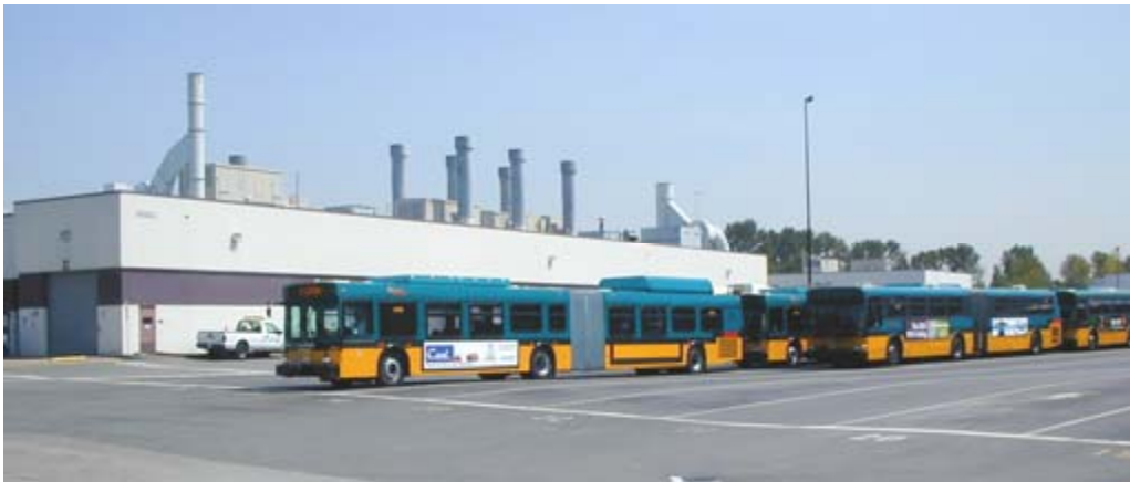
Figure 10. South Base Maintenance and Office Building
