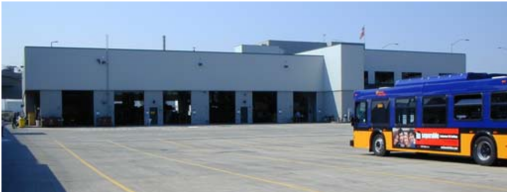
Figure 12. Ryerson Base Maintenance and Office Building
